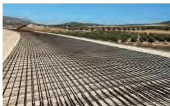
Continuous two-layer reinforced concrete pavement in the Yecla-Caudete section of the A-33 motorway, between Blanca and La Font de la Figuera
